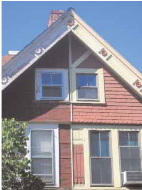
A Victorian house in Upham's Corner, a microneighborhood in Boston, demonstrates the gradual gentrification of both a building and a neighborhood. The perception of a neighborhood often lags behind the revitalization efforts of developers and real estate professionals.
